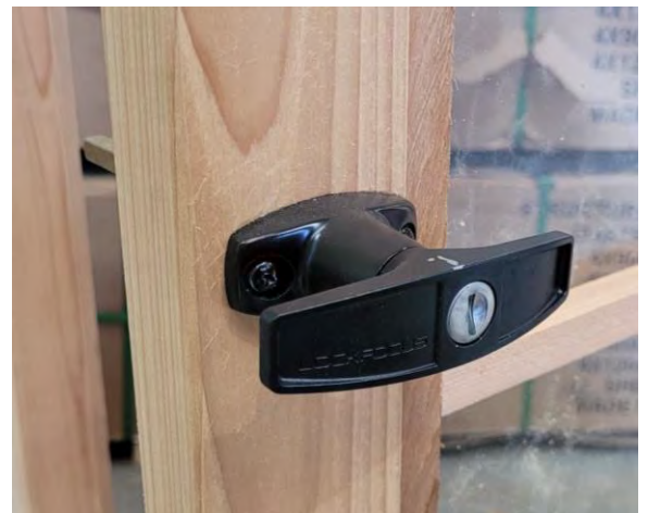
Drill 6mm holes and fasten t-handle to door with bolts, nuts, and washers.
