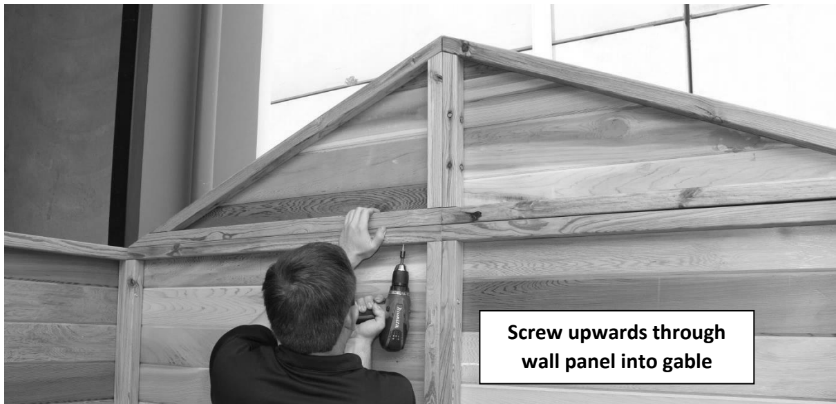
Ensure groove slots into tongue
